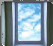
Skylight Above Tub/Shower
