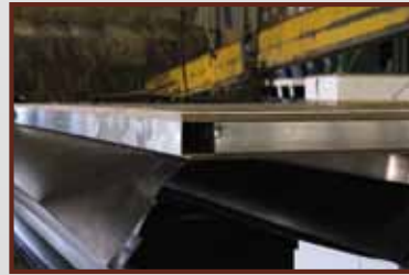
Aluminum Frame Floor and Side Wall Construction
