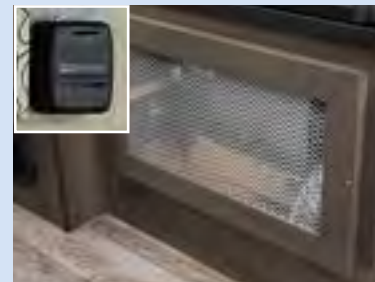
20,000 BTU Ducted furnace
