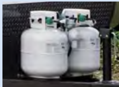
Double 20 lb. LP tanks
